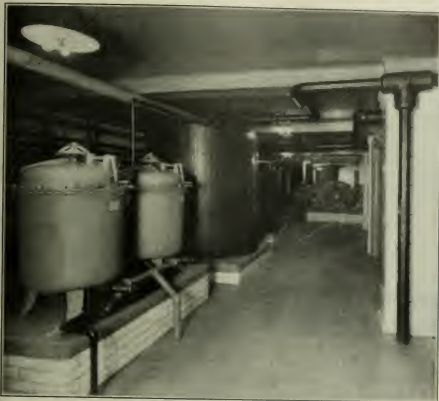
FIG. 15. WATER FILTERS, COOLING TANK AND VACUUM CLEANING APPARATUS
